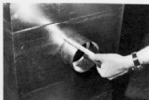
Figure H—Collar in duct min. 2"
