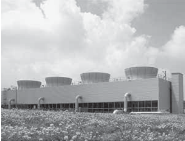
FIGURE B.1(d) Typical Induced-Draft Counterflow Water-Cooling Tower.
